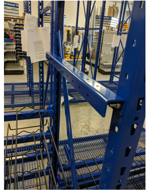
Mounted with bolt and nut
